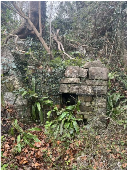
Figure 2. Gower's last surviving outdoor boiling cauldron, Pwlldu Lane, Bishopston
